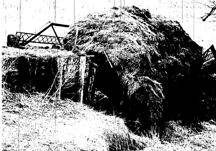
BRIDGE CLOSED — FULL OF HAY: This hay stack proved too much for a bridge six miles west and one and a half miles north of Wayne Saturday. Ray Agler was moving the stack for Monday morning the stack was removed by Milo Meyer but the damaged bridge will be closed until repairs can be made. Three nearby farmers, Sandahl, John Gathje and Herbert Niemann, all used the bridge to get to their fields.
